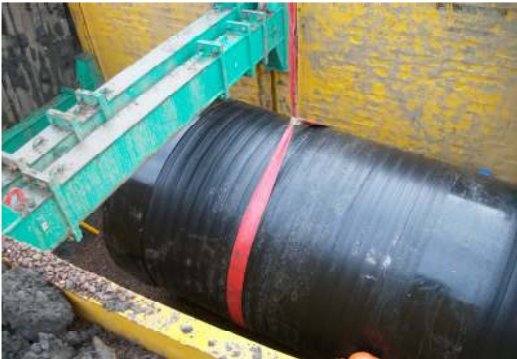
LAYING 2200MM PIPE
